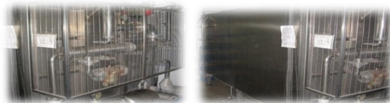
Figure 7. CIP cleaning standard of charging system
