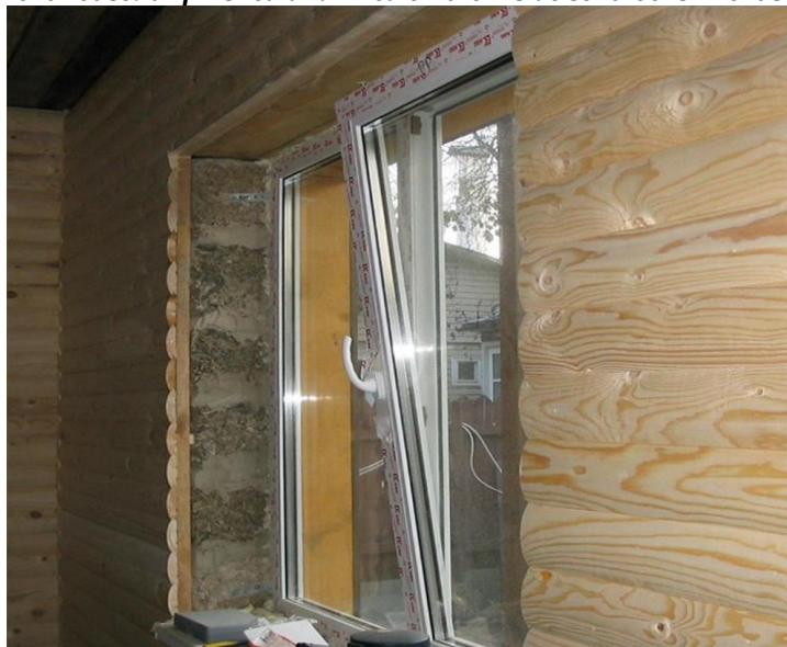
Fig. 6 Wood-cement house: unfinished and lined on the inside so it looks like it's built of wood. [3]
